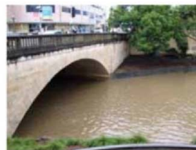
PHOTOS FROM 2011 HEAVY RAIN
