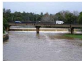
PHOTOS FROM 2011 HEAVY RAIN
